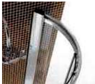
Aluminium cover profile (concealed fixings)
