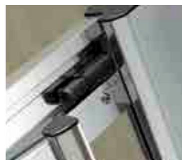
Spring loaded door buffer (on ALL sliding doors)
